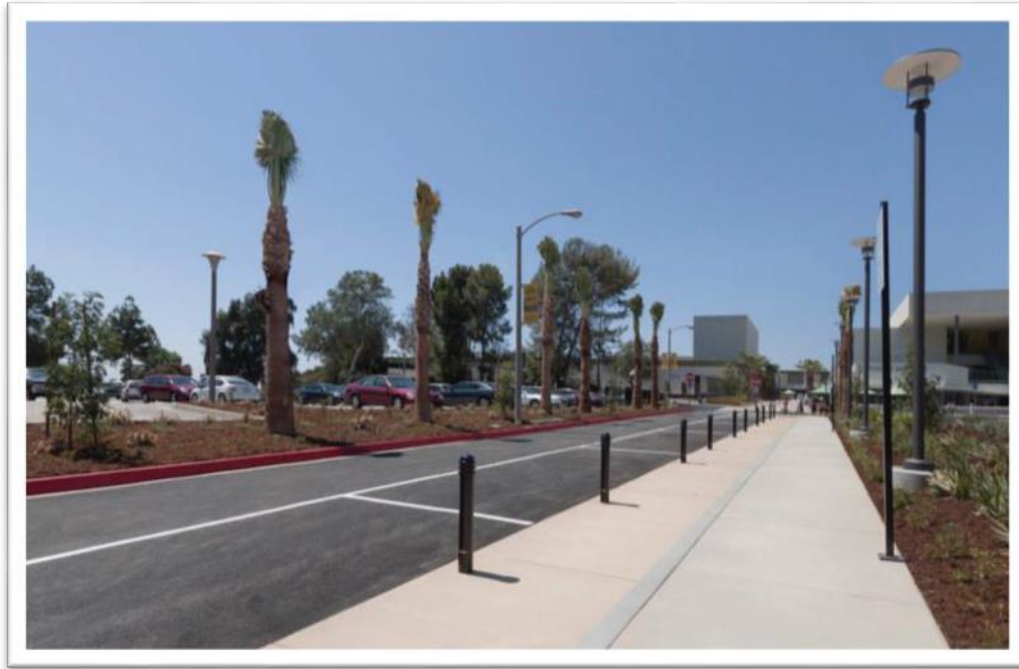
East Campus Vehicular Drop-off Completed: 2011
