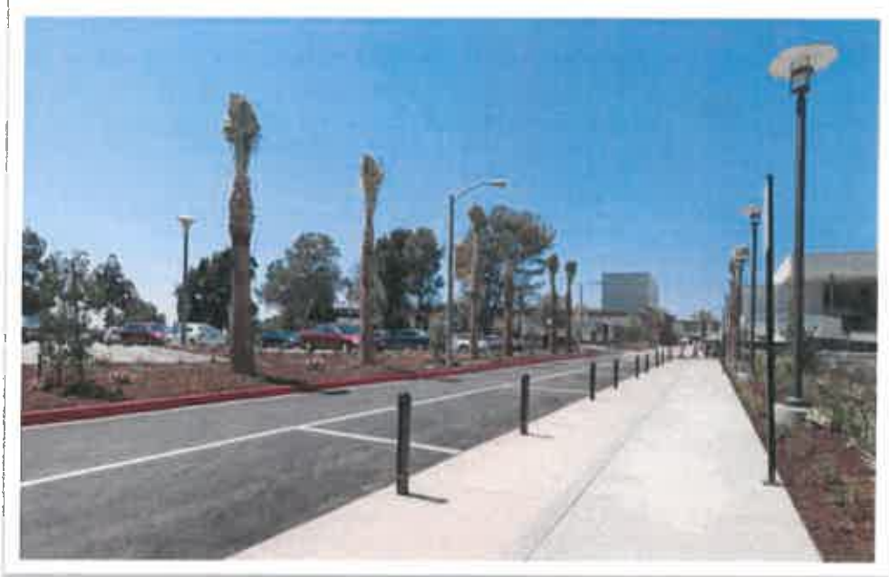
East Campus Vehicular Drop-off Completed: 2011
